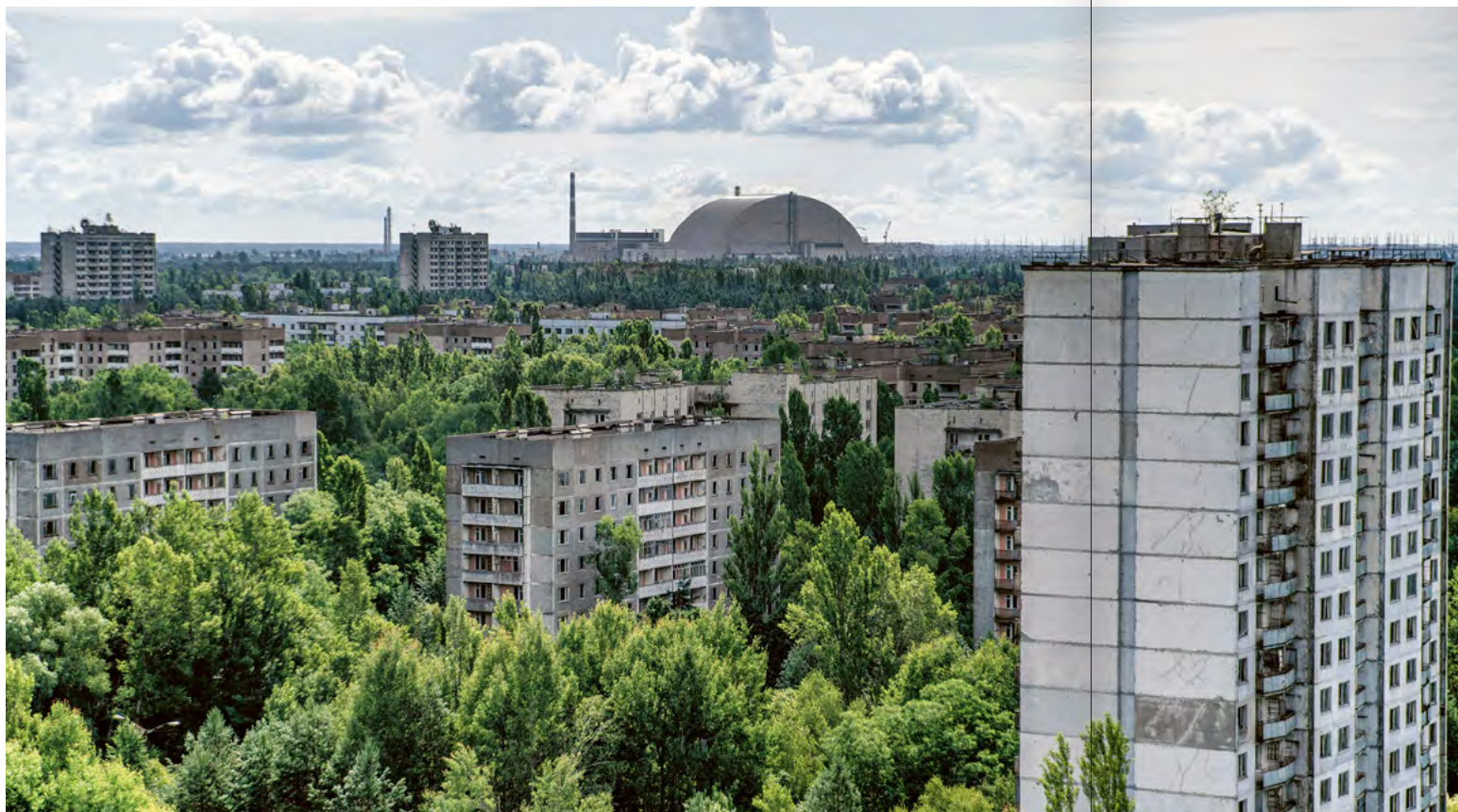
Figure 35 View from the top of an apartment complex in Prypiat, 2019. Courtesy of Carsten Olsen.
