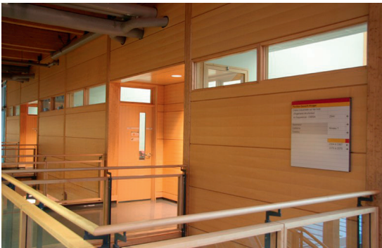
Figure 9.51 Example of intermediate partitions above head height, CTBO Pavillon, Laval University, Québec, Canada. Photo: Marie-Claude Dubois.
