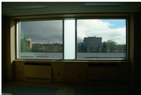
Figure 9.39 Effect of diffusing glass, Campus Laval University, Quebec, Canada. Photo: Marie-Claude Dubois.
