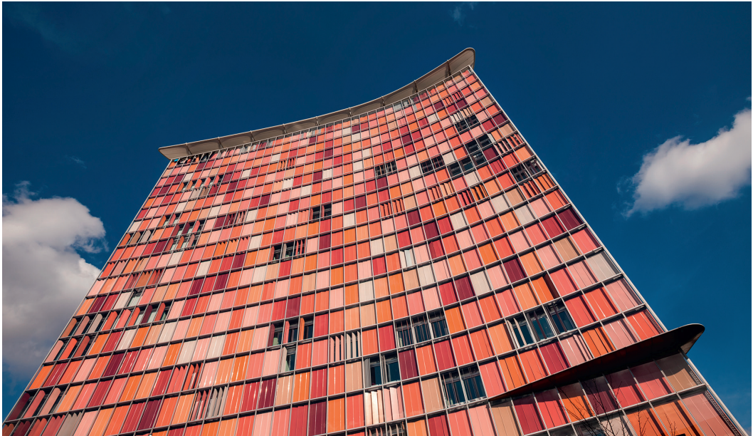
Figure 9.15 Rotating vertical slats for the east-west façade of the GSW building in Berlin. Photo: Michael von Aichberger/Shutterstock.
