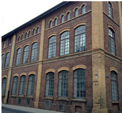
Figure 2.15 Typical factory building from the industrial revolution with large windows on lower floors, Cologne, Germany. Photo: Marie-Claude Dubois.
