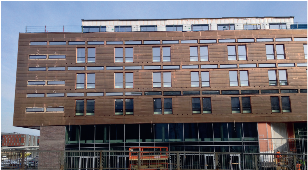
Figure 9.28 Example of a vision and daylight window (upper part) and its consequences on the expression of the façade. Trondheim, Norway. Photo: Marie-Claude Dubois.
