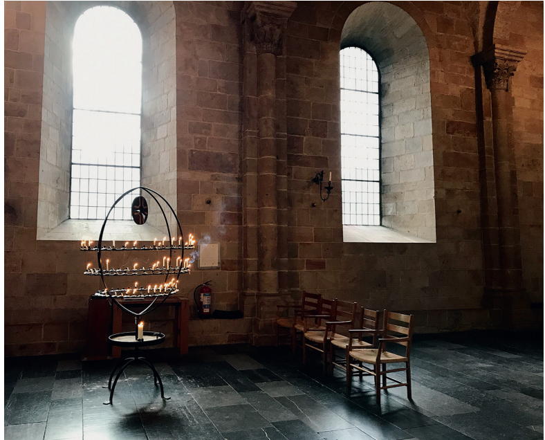
Figure 9.30 Example of windows in a load bearing construction, Cathedral of Lund, Sweden. Wall cavity around the window is splayed, which provides subdued contrast and better daylight penetration. Photo: Marie-Claude Dubois.
