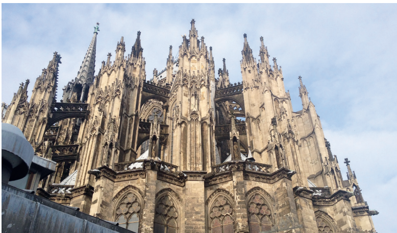
Figure 2.10 Flying buttresses at the Cologne Cathedral, Germany. Photo Marie-Claude Dubois.
