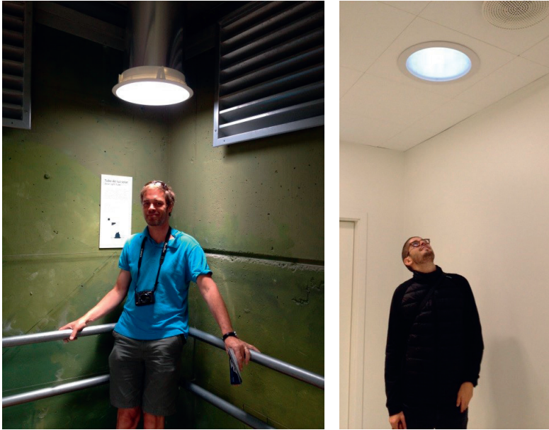
Figure 10.20 Tubular daylighting device under a sunny (left) and an overcast (right) climate. The picture on the right side shows a scene mainly illuminated by electric lighting.
