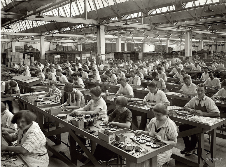
Figure 2.14 Sawtooth skylight illuminating factory workers during the industrial revolution. Photo: Everett Historical/ Shutterstock.com.
