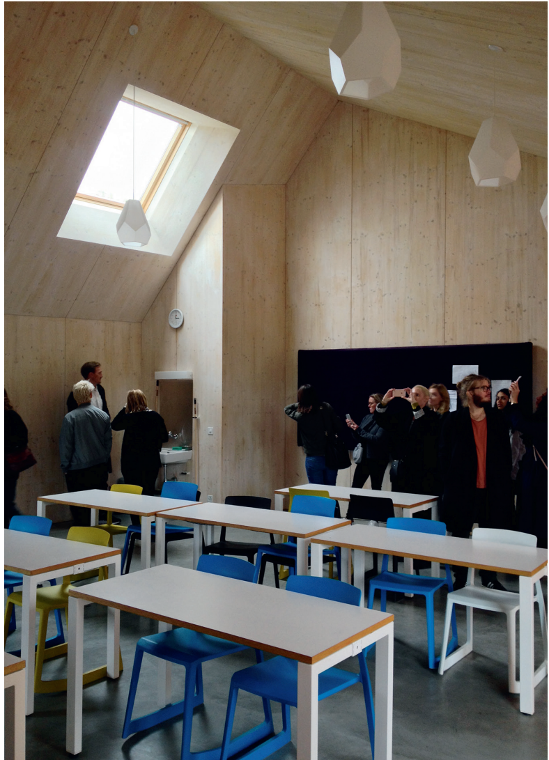
Figure 9.34 Splayed opening around the skylight of the Bois-Genoud school in Lausanne, Switzerland, by Localarchitecture. Photo: Marie-Claude Dubois.
