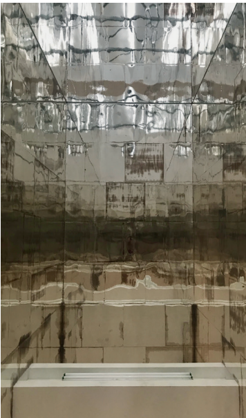
Figure 10.19 Light wells of the National Gallery of Canada, Ottawa, Ontario, Moshe Safdie, architect. The image on the left shows the highly reflective surfaces used inside the light wells.
