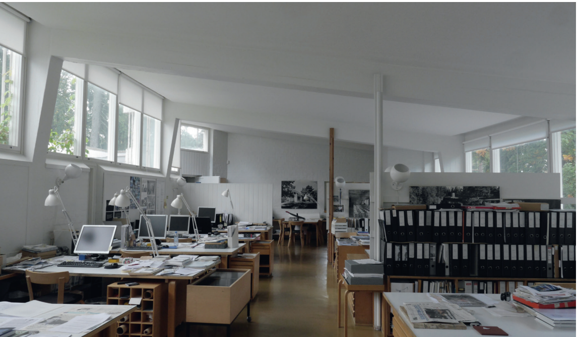
Figure 9.25 Example of high window position for good ambient daylighting, Alvar Aalto studio, Helsinki, Finland. Photo: Malin Alenius.
