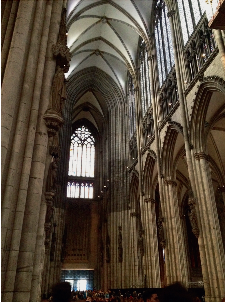
Figure 2.9 Cologne Cathedral, built 1248-1473, Cologne, Germany, showing the pointed ogival arch and the ribbed vault. Photo: Marie-Claude Dubois.
